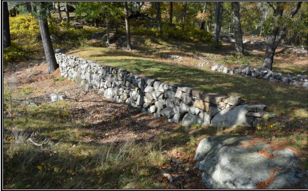
The western portion of the Marine Battery, facing northwest; the stone work in the foreground is the revetment (stone face) for the battery's parapet base / rampart; the line of stones to its right is the cannon platform base (Panamerican 2016).
