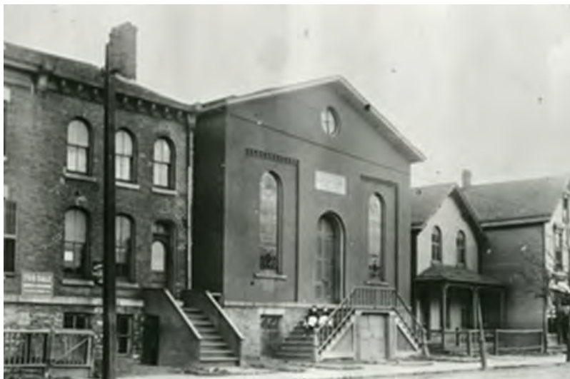
Street-view of 515 Michigan Avenue and the southern part of 517 Michigan Avenue, owned by Peyton Harris (foreground-left), and the Michigan Street Baptist Church at 511 Michigan Avenue (foreground at right). This undated photograph was likely taken between c. 1898-1908. Courtesy of Buffalo Historical Museum.
