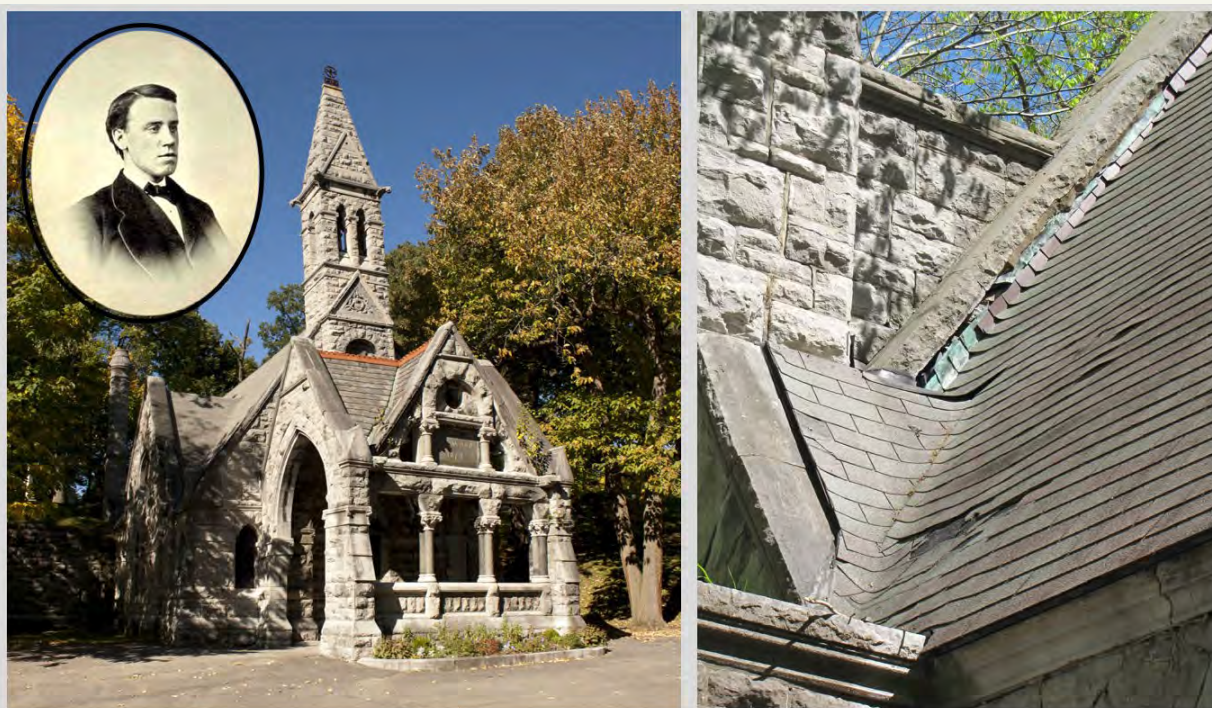
Fig. 5. Designed by architect Joseph Lyman Silsbee (upper left) , the mortuary chapel was built in 1879. Over the years the roof joints deteriorated and water was entering the building. To alleviate the problem, flashing at the gable joints was replaced in 2021.
