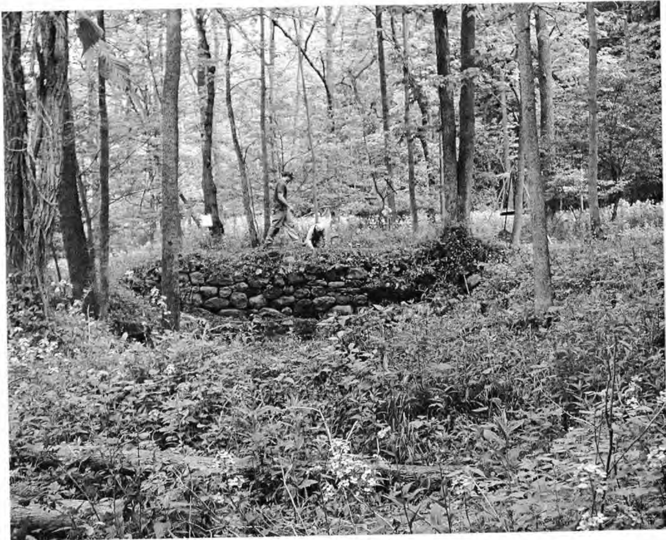
Figure 12. Dixon House foundation, c. 2004, looking toward north side of house after clearing.
