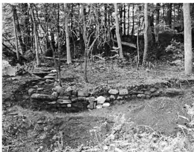
Figure 19. Grove Mather House foundation, view looking north.
