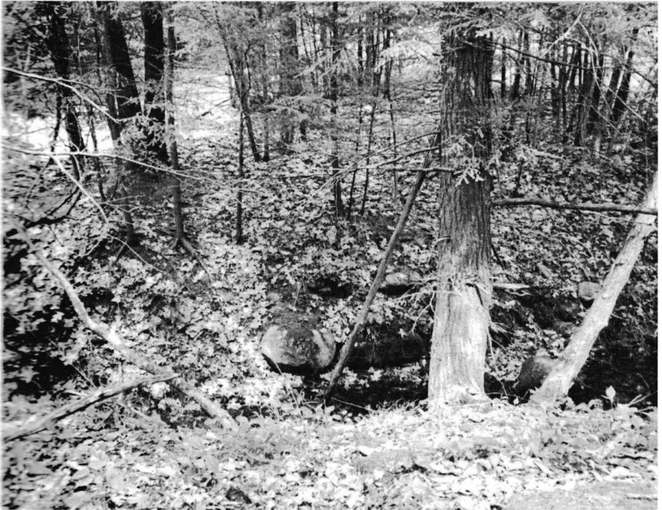
Figure 9. View of Adams' Mill foundation, view looking north and toward the outlet.
