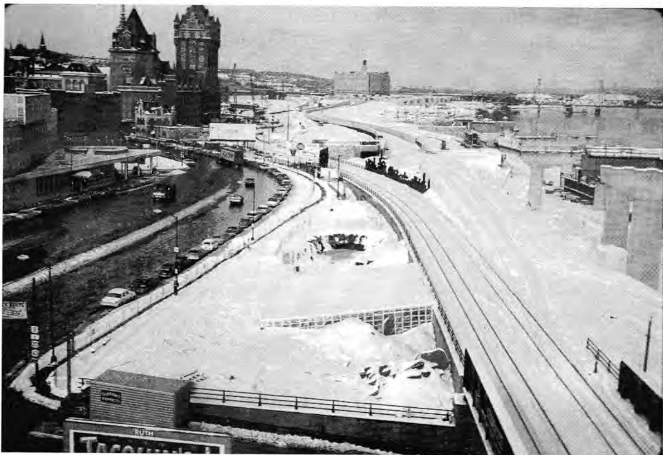
Figure 2. View northward from the new Hudson River bridge of the site after the first snowstorm, December 1970.
