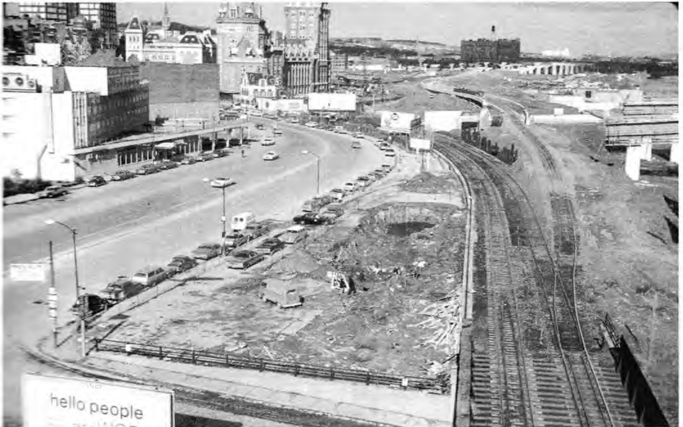
Figure 1. View of the initial test excavation northward from the new Hudson River bridge, November 1970.
