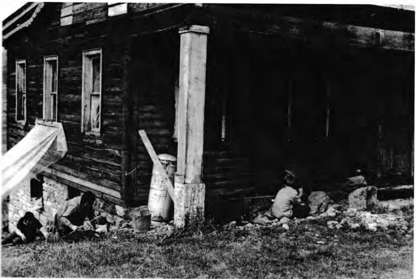
Figure 4. Schoharie Crossing canal store excavations, 1976.
