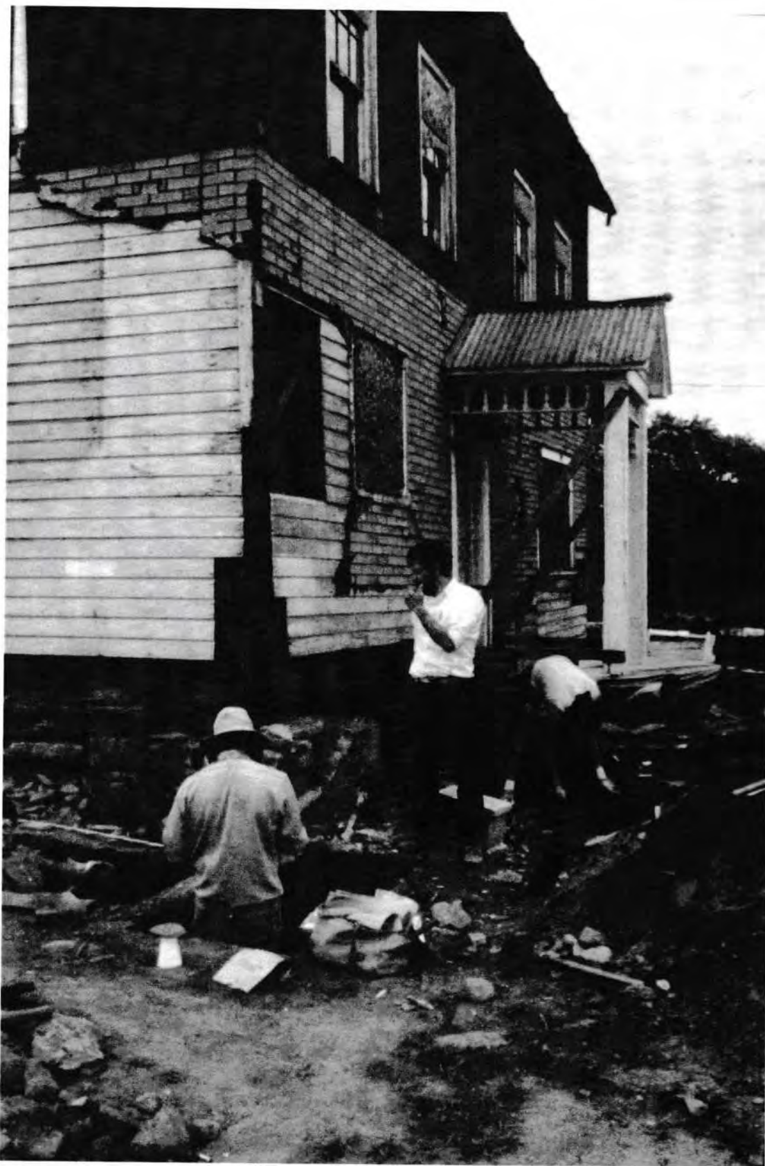
Figure 5. Enders house excavations, 1990.
